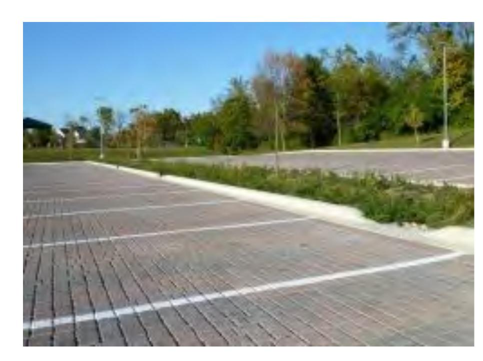
Permeable pavement in the parking lots will reduce a lot of runoff. Along with this, planting vegetation along the daylighted river and the lower portion of the building will reduce chances of erosion and flooding. All while adding an aesthetic appeal. Since the largest building's lower section is prone to flooding, adding these features will reduce flooding as well as acidic runoff.
